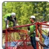
Dismantle scaffolding up and clean up
