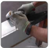
Joining- knock up joint
