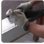
Joining- knock up joint
