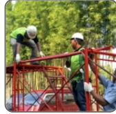
Dismantle scaffolding up and clean up
