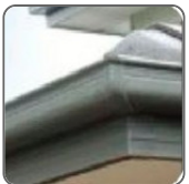
an eaves gutter
