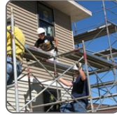
Inspect, repair and alter scaffolding
