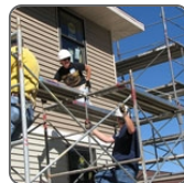
Inspect, repair and alter scaffolding
