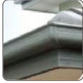
an eaves gutter
